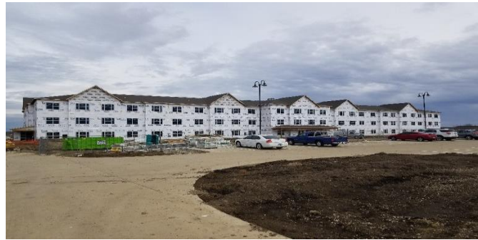
Picture 9 - Haven Court Under Construction
