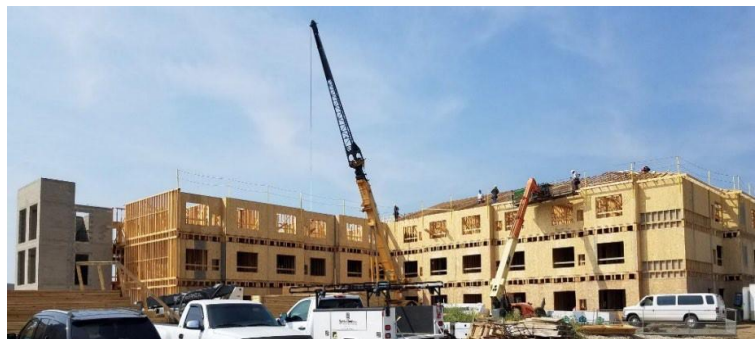
Picture 2 –The Haven at Market Place Under Construction
