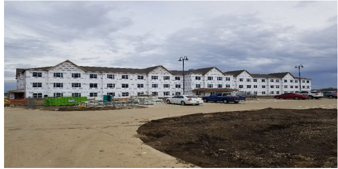
Picture 9 - Haven Court Under Construction
