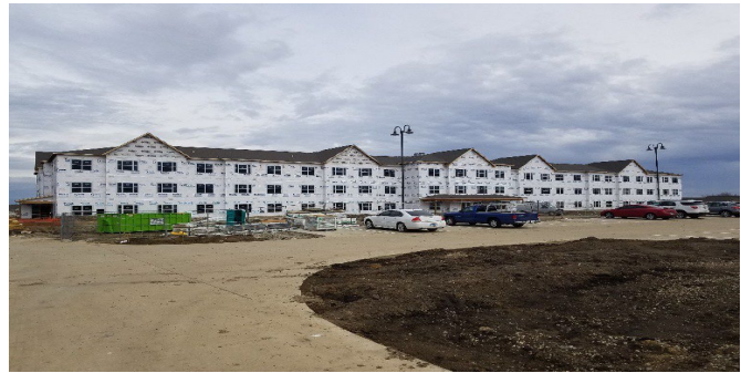
Picture 11 - Haven Court Under Construction
